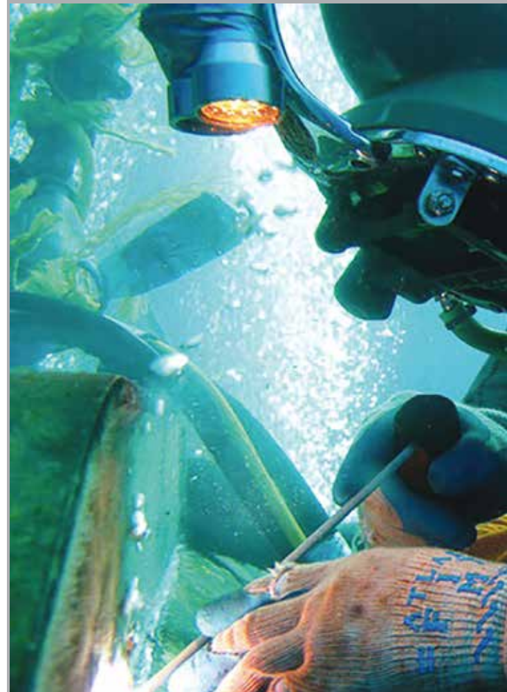
UNDERWATER BURNING AND CUTTING
