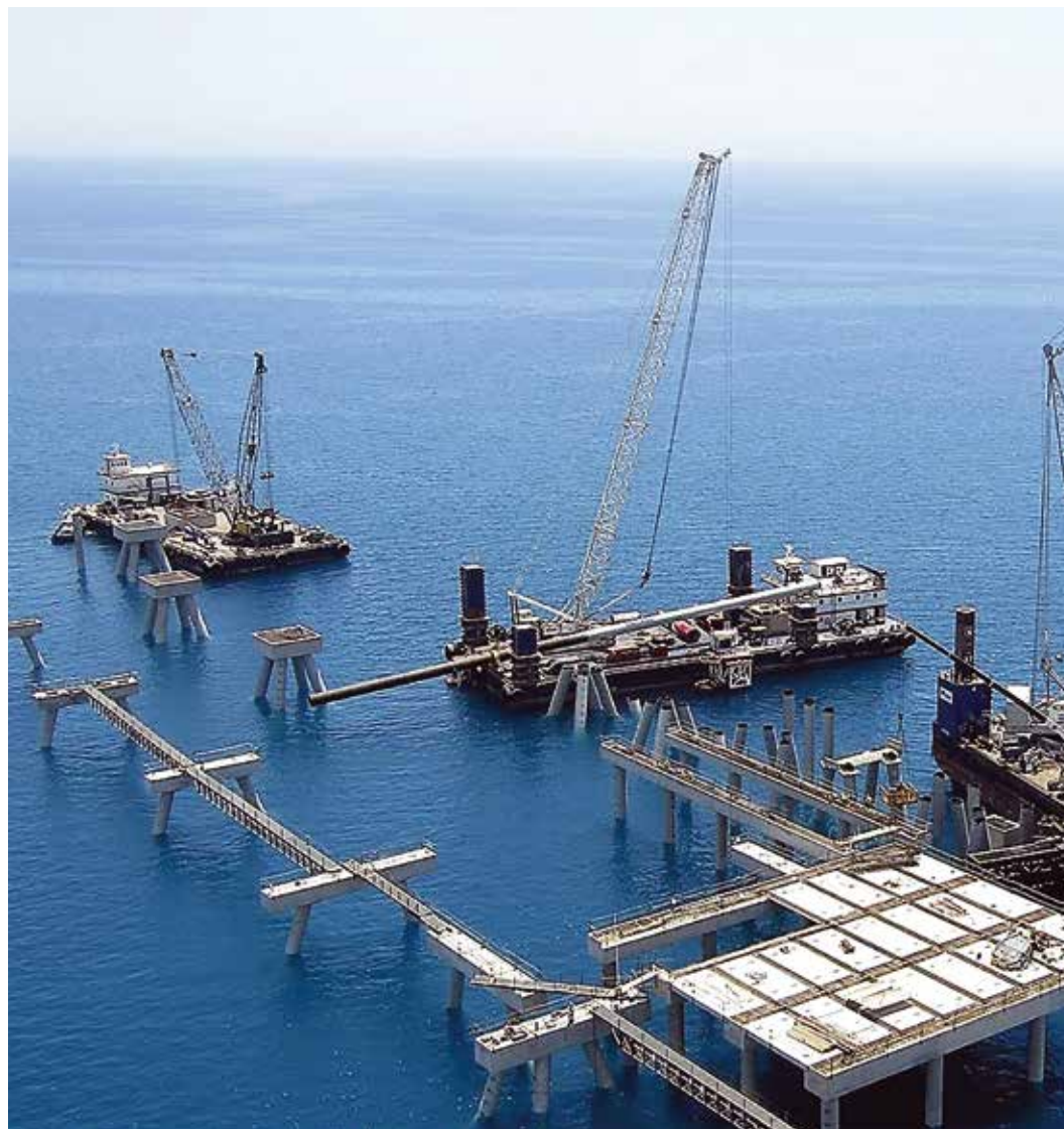
JETTY'S PLATFORM ERECTION
