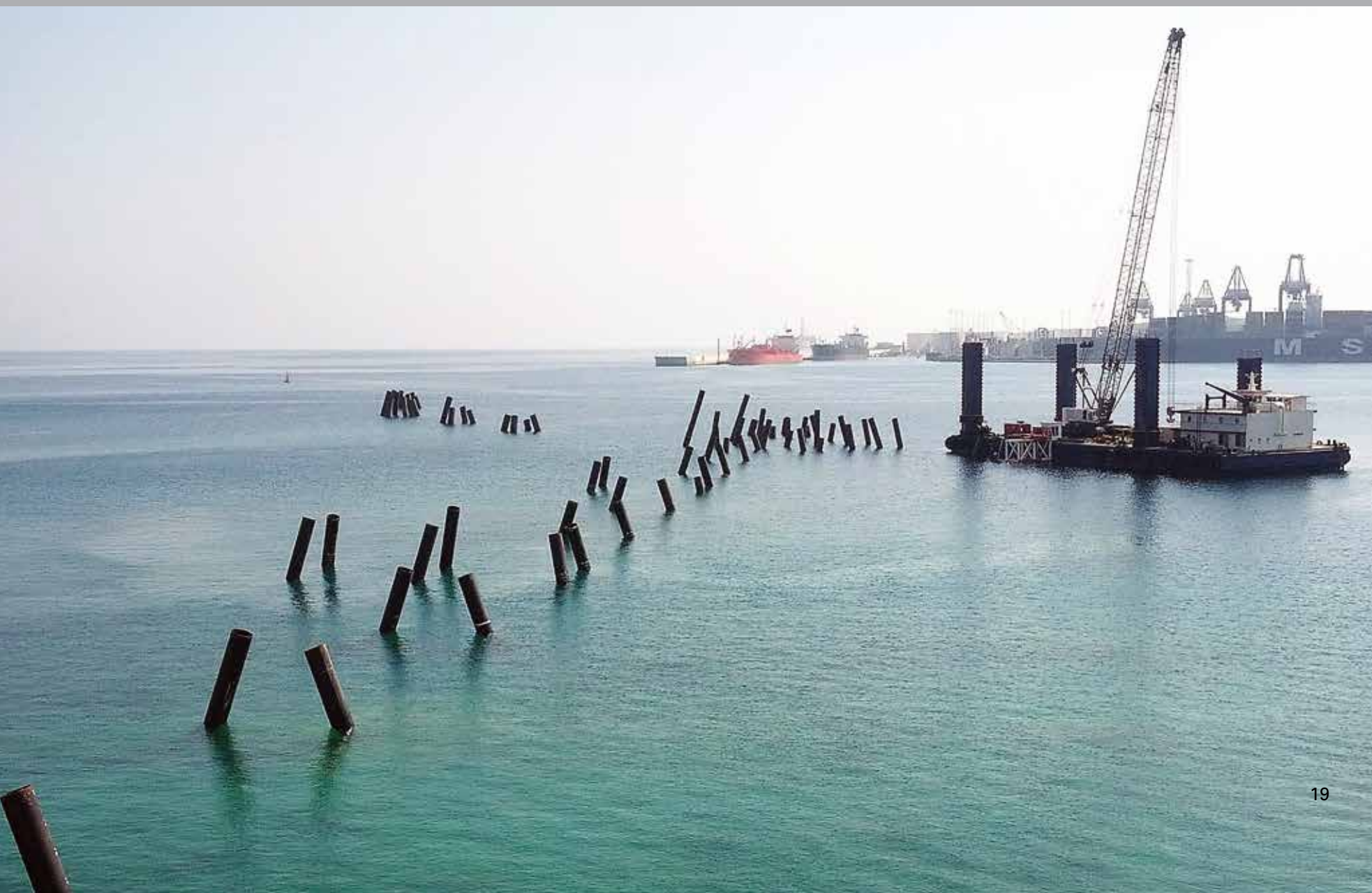
DRIVING OF STEEL PILES
