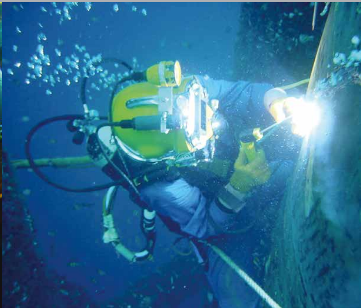
UNDERWATER WELDING FOR SALVAGE OPERATION
