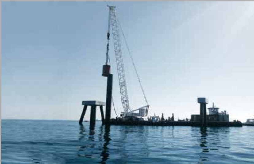
MONOPILES INSTALLATION
