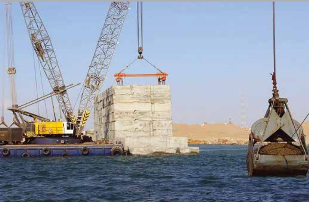
QUAY WALL CONSTRUCTION
