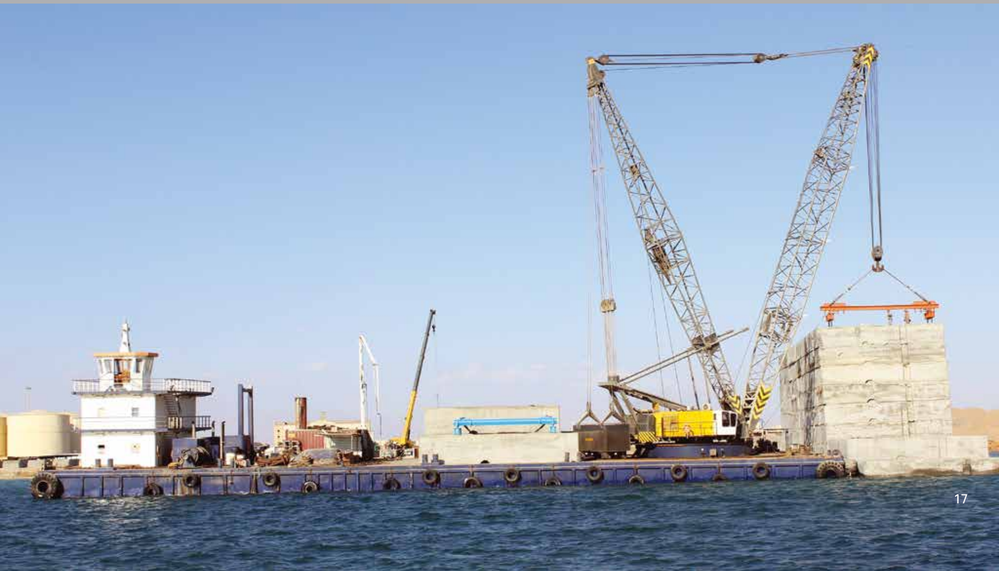
CONCRETE BLOCKS LAYING
